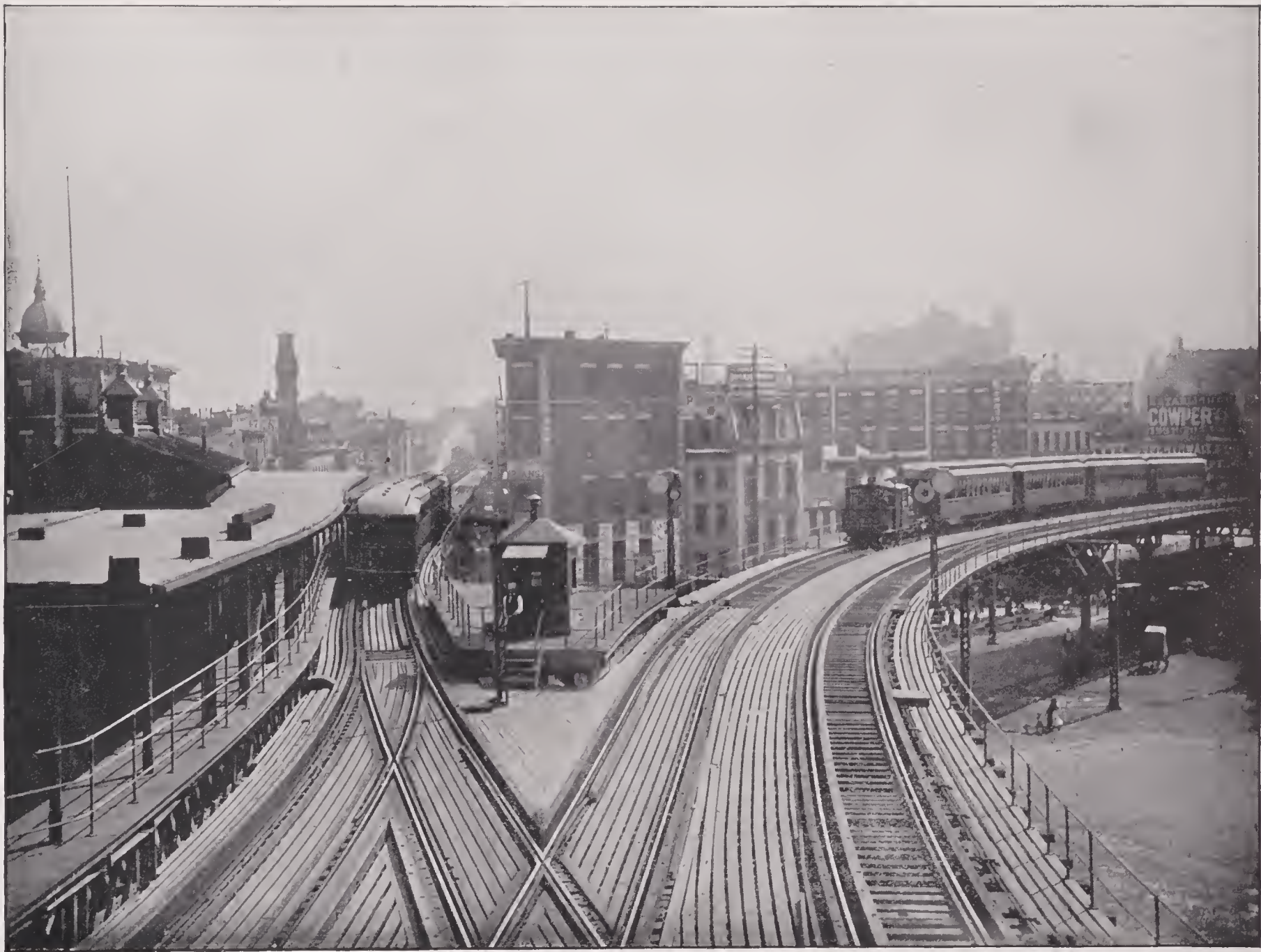
ELEVATED RAILROAD, NEW YORK CITY, N. Y.—The steam cars, the street railway and the electric road are the three modern modes of transportation. The motive power of the elevated railroads of New York City is steam, and the quick facilities afforded exceed that of any other country. These elevated railroads are sufficiently high so as not to interfere with street traffic, stations are located every four or five blocks apart, there is little delay, and a passenger can ride from one end of the city to the other in a very short time. It is said that one million people ride daily on the elevated railroads of New York, giving the company an income of $50,000 per day. The above photograph represents the railroad at Chatham Square, where it branches off into different directions.
